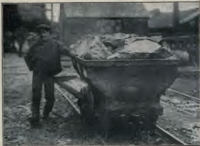
A MINE CAR LOADED WITH COAL.
